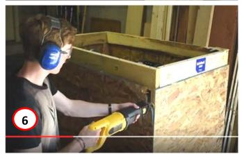
**6)** Continue with the crowbar or use a sawz-all to remove the rest of the crate. Be sure to wear your personal protection for eyes and ears.
