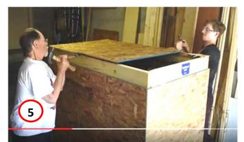
**5)** The crate is assembled with lots of ring-shank nails. Your first step should be to pry off the top and have a look at the layout inside.
